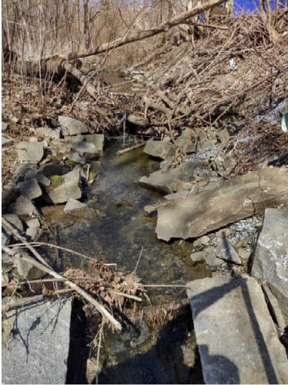
FACING NORTH, APRIL 2022
