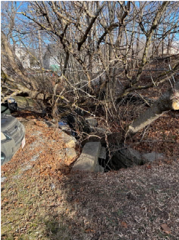
FACING NORTH-EAST, DECEMBER 2020
