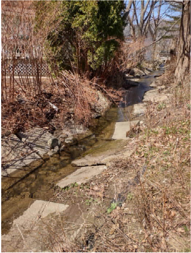
FACING NORTH-WEST, APRIL 2022
