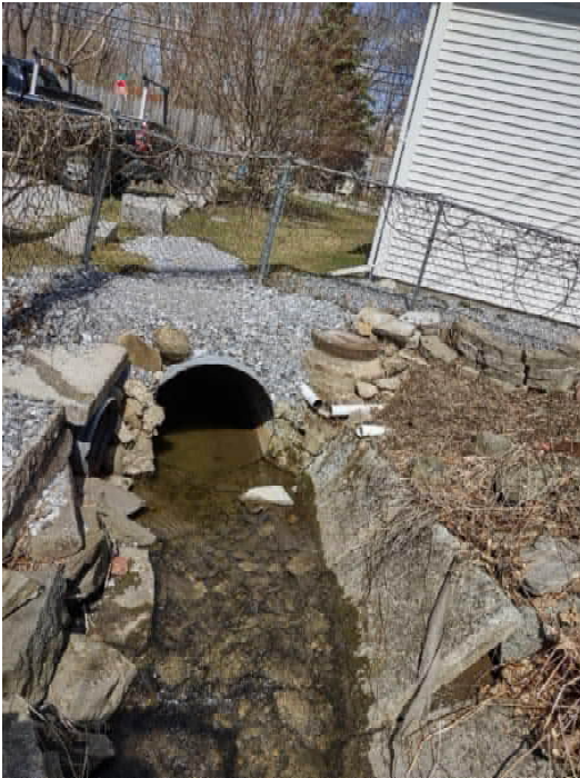
FACING NORTH, APRIL 2022
