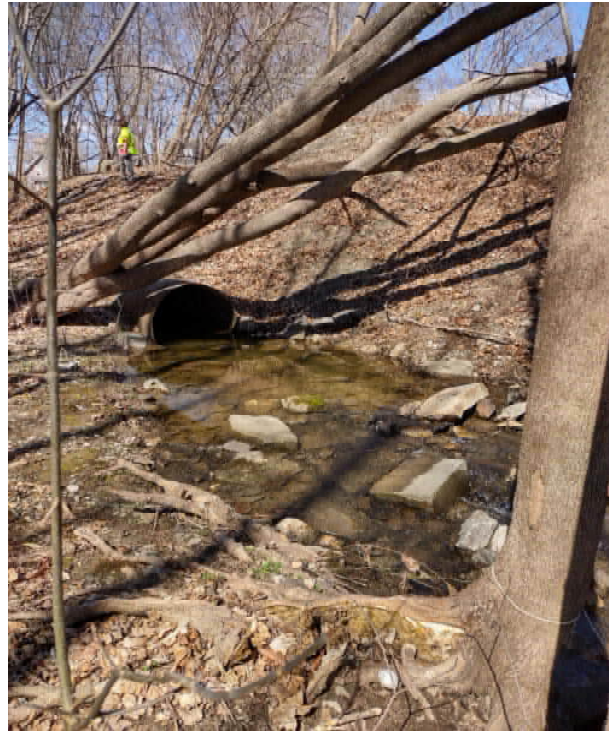
FACING NORTH-WEST, APRIL 2022
