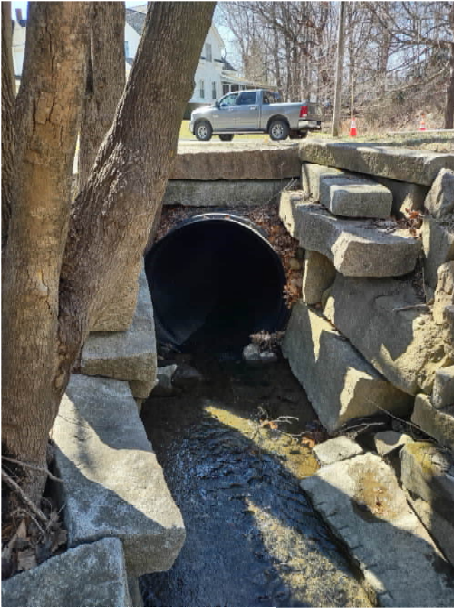
FACING SOUTH-EAST, APRIL 2022
