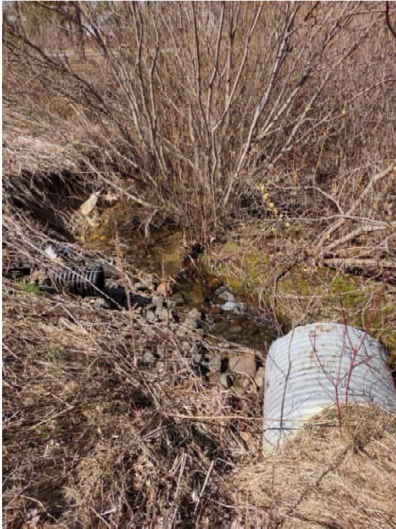
FACING NORTH, APRIL 2022
