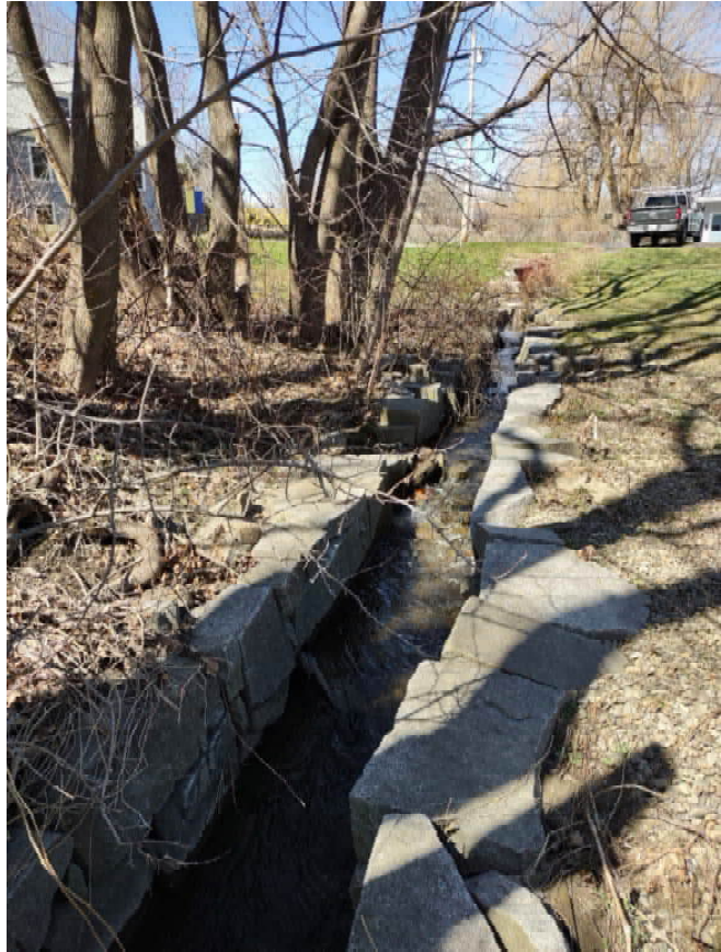
FACING NORTH, APRIL 2022
