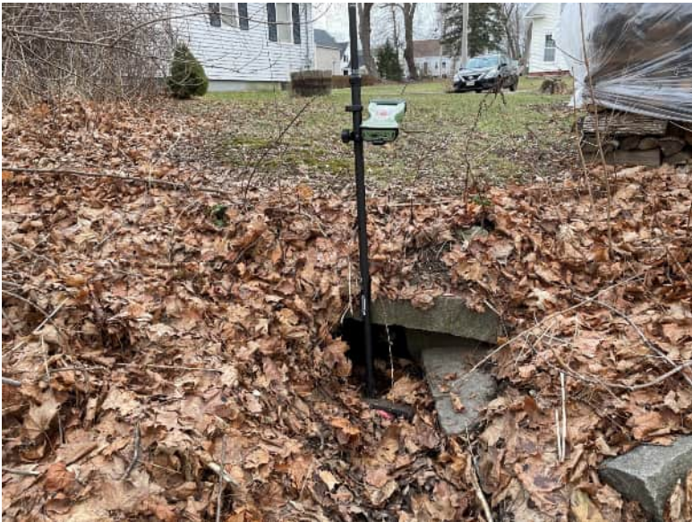
FACING SOUTH-WEST, DECEMBER 2020
