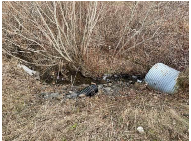
FACING NORTH-EAST, DECEMBER 2020
