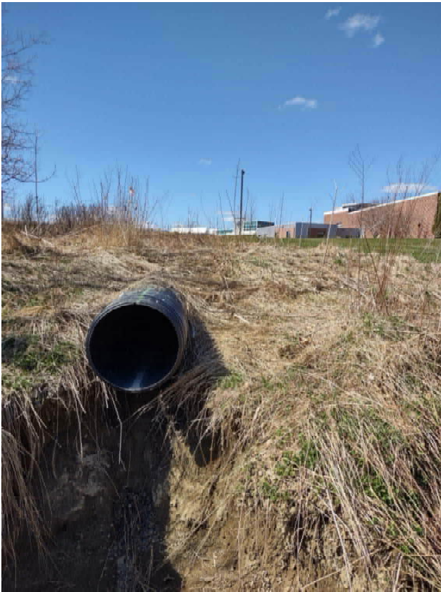
FACING NORTH-WEST, APRIL 2022
