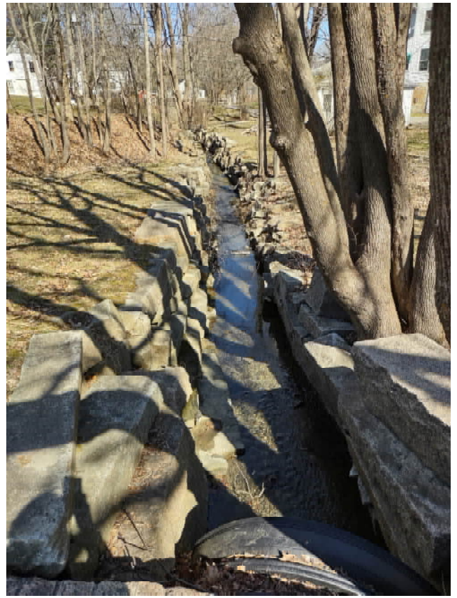
FACING NORTH, APRIL 2022
