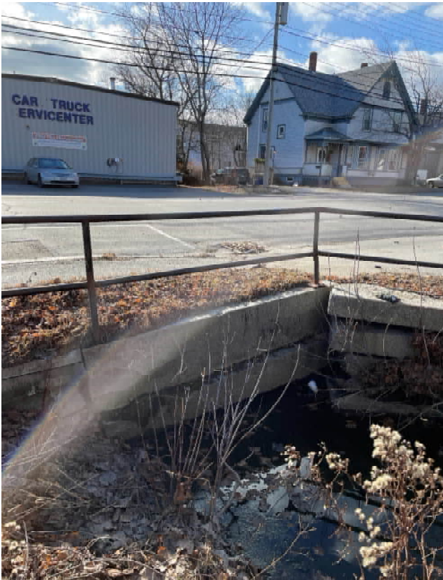
FACING SOUTH-WEST, DECEMBER 2020
