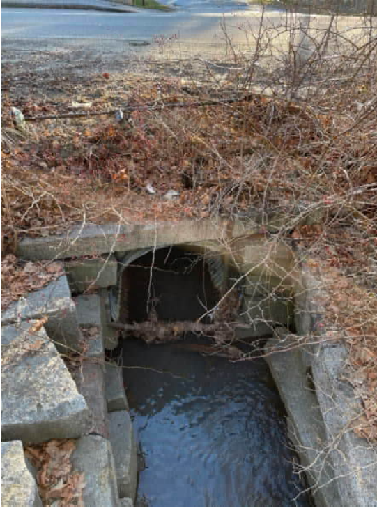
FACING SOUTH-WEST, DECEMBER 2020
